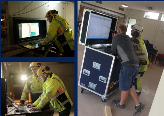
Example of BIM stations on- site
